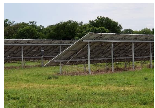
Example of a Solar Conversion System, Ground-mounted
