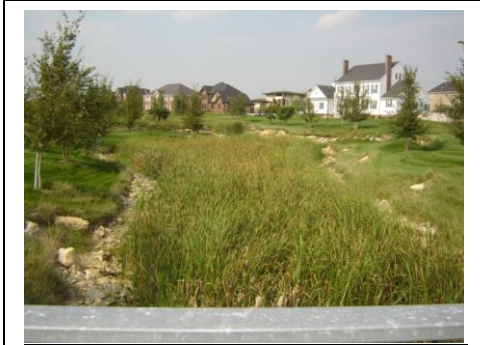
Example of a Drainageway or Surface Drain
