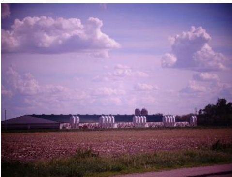
Example of an Animal Confinement Building
